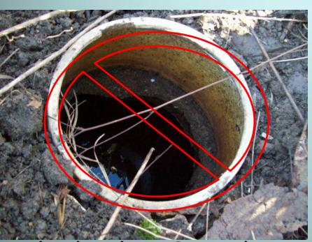
...the bucket & trash can lid over the tank opening is a safety hazard--especially for children.
