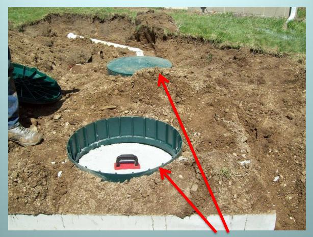
An example of a proper septic tank riser. Note the riser lid extends to the ground surface & there is a manhole cover over the septic tank opening.
