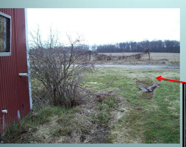
Pictures showing the open hole from the collapsing septic tank
