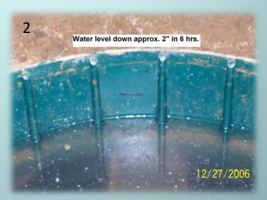
(Pictures are showing a septic tank riser with the lid off.)
