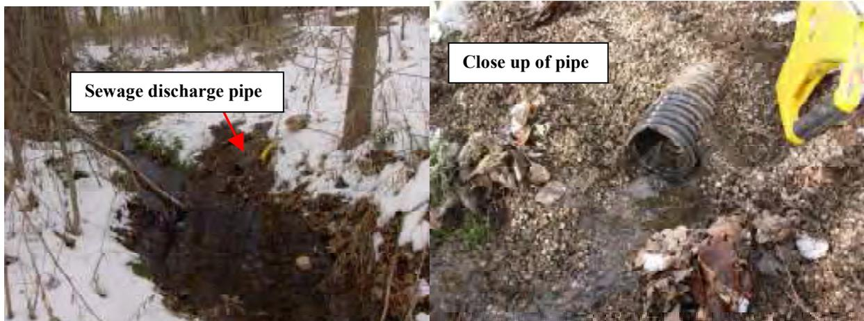
The two pictures above were taken by a registered evaluator and identify a bleeder line (illicit connection). The line runs approximately 125 feet from the septic tank to this creek. This creek is a tributary of the Coldwater River which is a trout stream but also has been identified by the MDEQ as a TMDL stream, which means fecal coliform bacteria exceed the daily maximum load for human contact.
