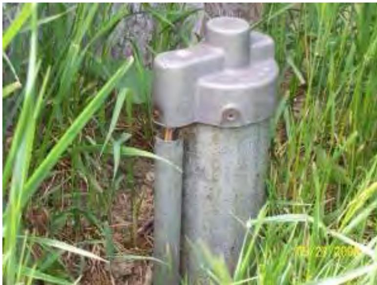
The above picture was taken by a BEDHD Sanitarian and shows a well cap with exposed electrical wires and the well cap screws had been removed. The cap could easily be removed. The hazard was corrected.
