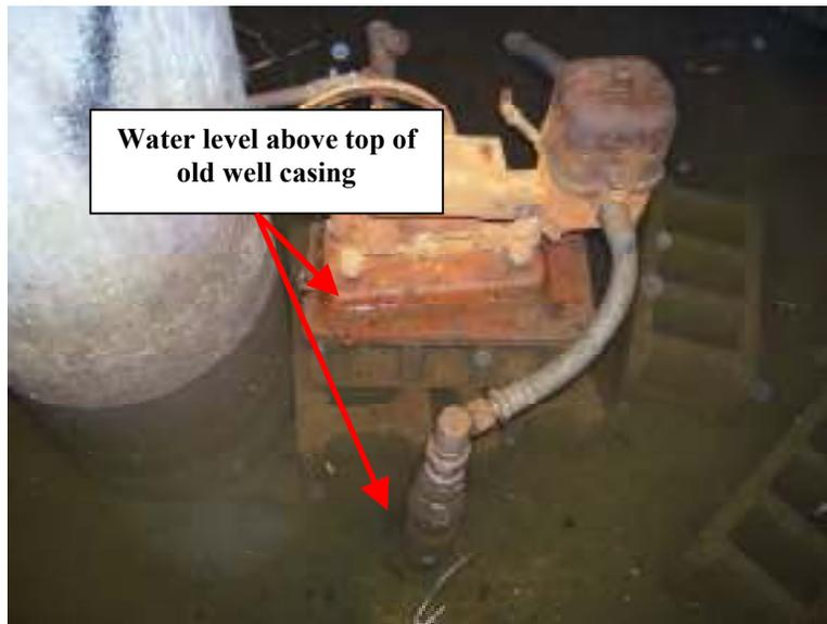
The above picture was taken by BEDHD Sanitarian and draws attention to an unplugged abandoned well in a flooded pit. Note the water level is just above the well casing of the unplugged well. Correction involved plugging of the old well by a licensed well driller.
