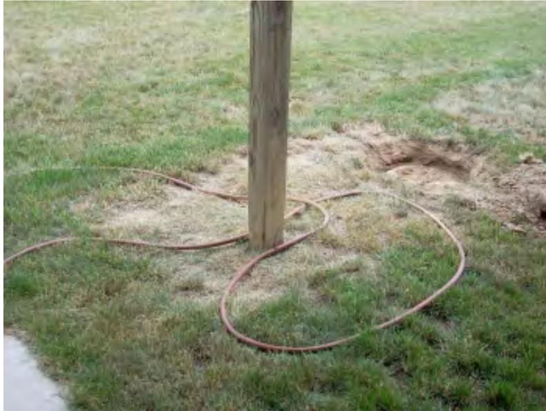
The above picture was taken by a BEDHD Sanitarian this year during a confirmation visit for TOST. The picture shows the corner support post of a large wooden deck that was installed on top of a septic tank. The deck post was re-located avoiding the collapse of the septic tank and potential simultaneous collapse of the large deck
