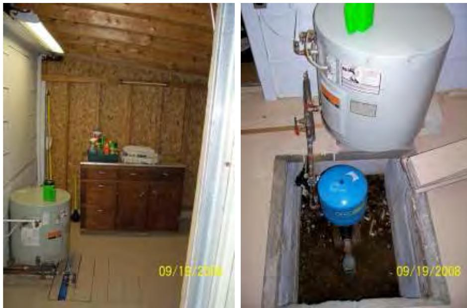
The above pictures were taken by a BEDHD Sanitarian this year during a confirmation visit for TOST. The pictures identify a well pit inside a structure. By building a structure over the top a well, access to perform work on the well is limited. While this situation didn't require correction prior to transfer, when this well is no longer in working order proper plugging will be more difficult to accomplish.
