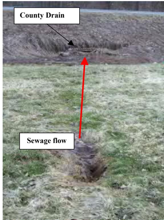
The above picture taken by a BEDHD Sanitarian and identifies a bleeder line installed to bypass the failed drainfield. The sewage was discharging on the ground surface and flowing to the County drain (identified at the top of the picture). A new sewage system was installed.
