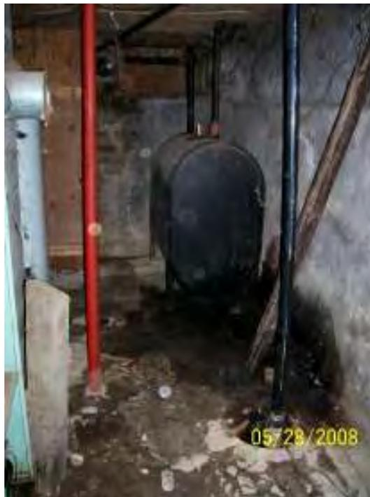
The above picture was taken by a BEDHD Sanitarian this year while performing a confirmation visit for TOST. The picture reveals a leaking fuel oil tank located in a basement. The fuel oil had been leaking and draining to a sump pump pit located in the foreground. The sump "water" was surface discharging. The drinking water well was located 35' away in a pit, outside the home. A new fuel oil tank was installed and properly isolated from the well.
